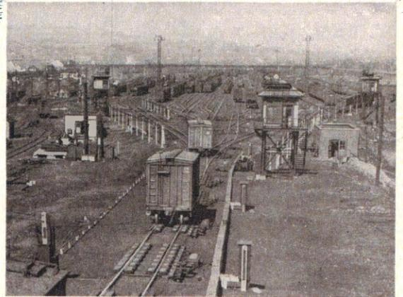
**CAR RETARDERS IN USE:** These modern machines controlled from central towers, exert pressure against the sides of passing car wheels to control their speed as they roll down the hump, and so expedite classification with smooth, shock-free switching.
